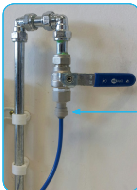
C) 1. A potable water source 2. A 1/4" push-fitting on the outlet
