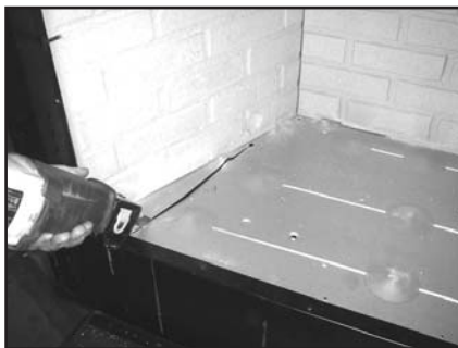
Figure 12.2. Using a saws-all, cut out the floor.
