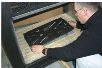
Diagram 1: Remove the left and right screws and then slide the burner assembly away from the orifice and lift out.
