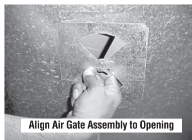
Figure 12 - Position Air Gate
