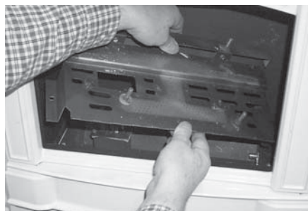
Pilot assembly is now accessible for steps 4) to 9).
