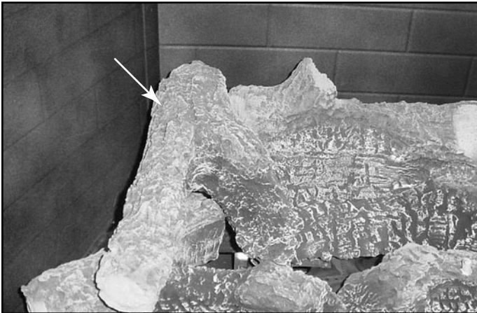
Figure 14.6 Placing Left Top Log
