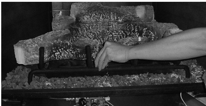
Figure 14.2 Placement of Vermiculite
