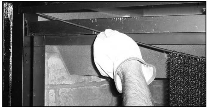
Figure 14.15 Insert Rod Into Side Columns
