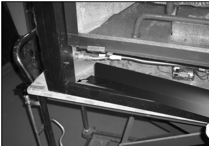
Figure 14.13 Installing Floor Cover
