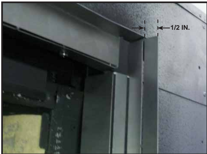
Figure 13.4 Finishing Templates Bends - Inoperable (Fixed) Doors
