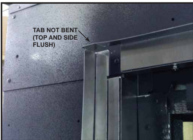
Figure 13.5 Finishing Template Bend - Operable Doors
