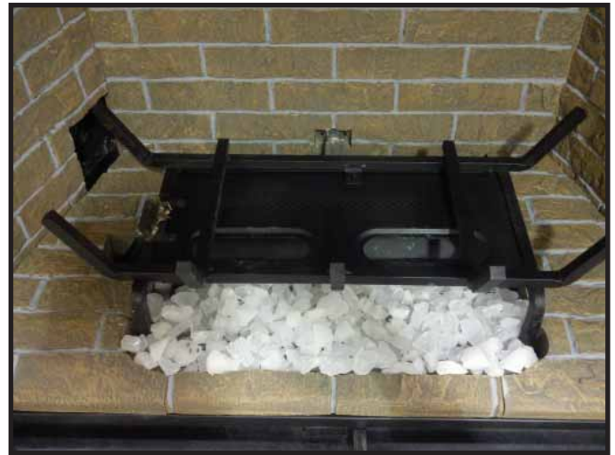
Figure 14.2. Ember Glass Area Covered with Teco-Sil
