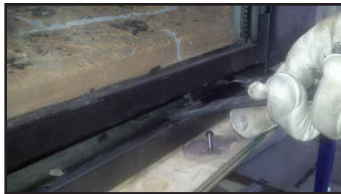
Figure 14.7. Glass Clip Tool Location
