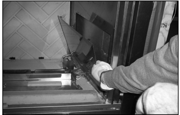
Figure 12.4 Remove Valve Access Panel
