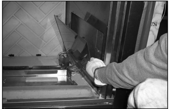
Figure 6.4 Remove Valve Access Panel
