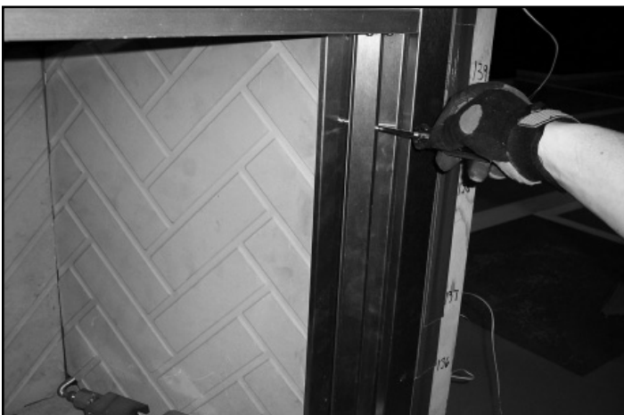
Figure 12.3 Loosen Refractory Retaining Strip
