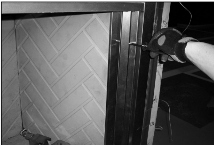
Figure 6.3 Loosen Refractory Retaining Strip
