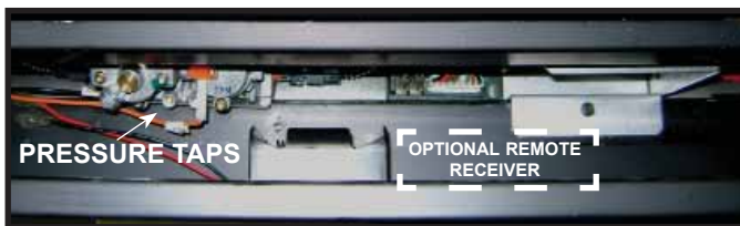
Figure 11.5 Valve Pressure Taps and Remote Receiver Location
