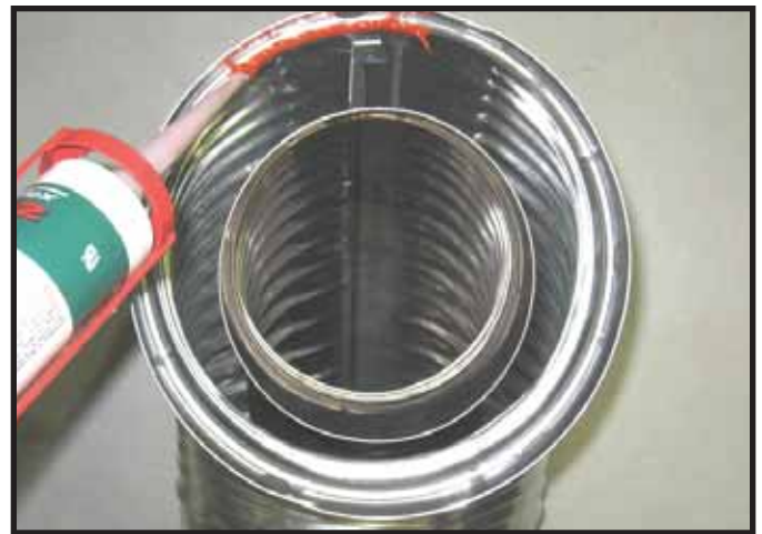
Figure 10.2 High Temperature Silicone Sealant
