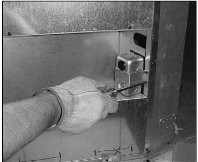
Figure 13.2 Remove Two Screws From Bracket
