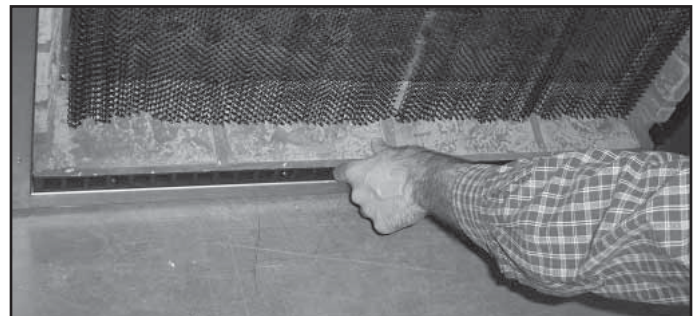
Figure 15.22 Placing Bottom Front Hearth Refractory
