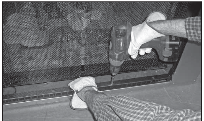
Figure 15.16 Install Lower Decorative Front Face
