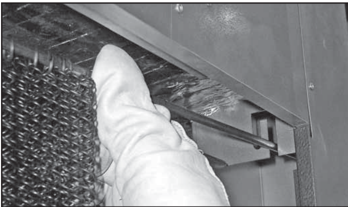
Figure 15.12 Place Right End of Screen Rod
