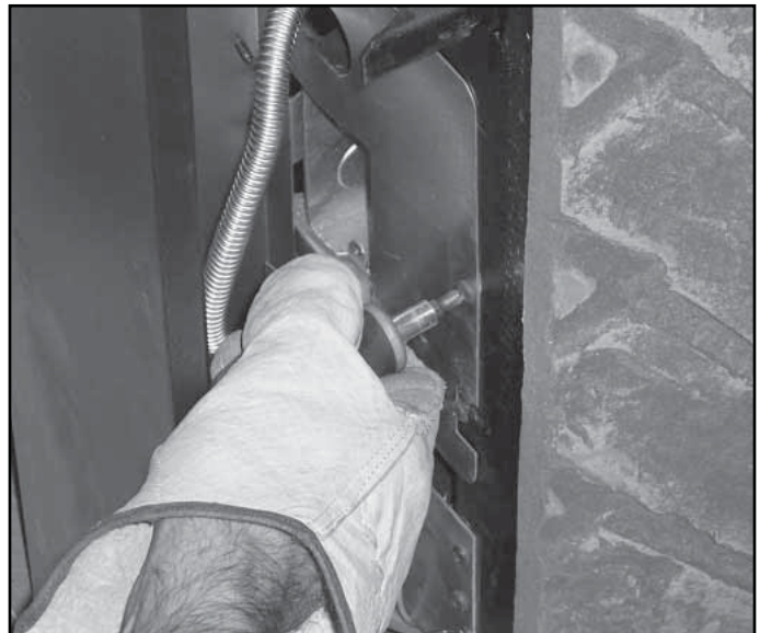
Figure 13.3 Remove Access Panel Screw
