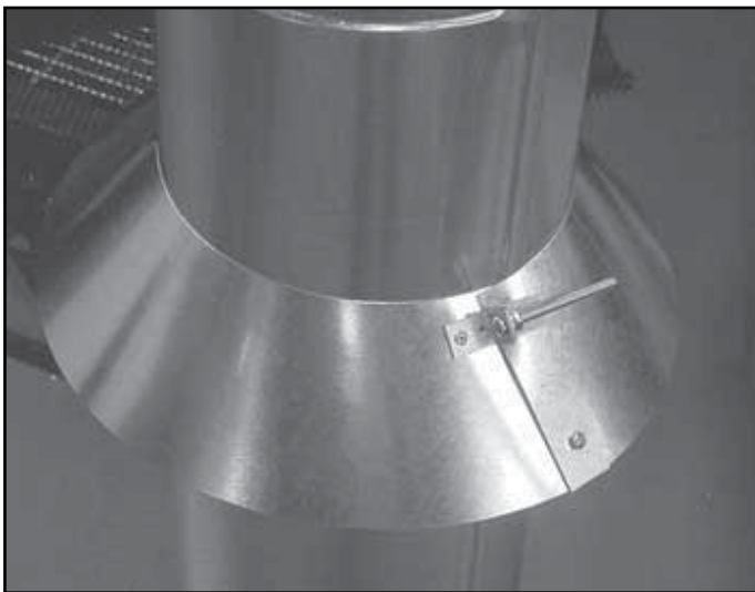
Figure 10.14 Assembling the Storm Collar Around the Pipe
