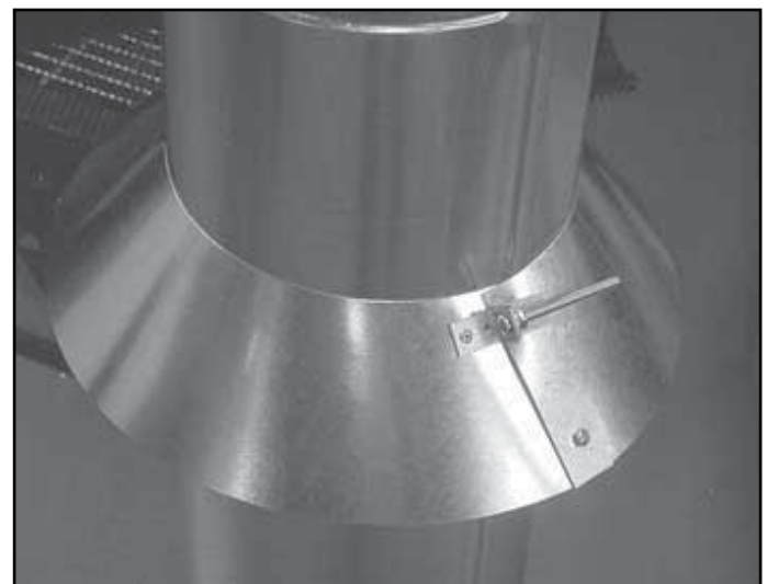
Figure 10.17 Assembling the Storm Collar Around the Pipe
