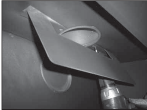
Figure 7.7a Remove Flue Visor
